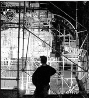
The scaffolding needed to restore the original fir ceiling.
